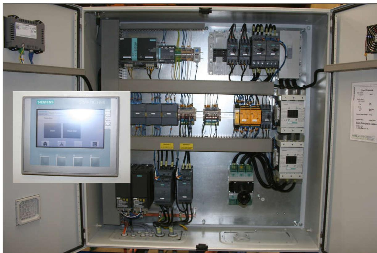
The control cabinet. Insert : The HMI-unit.
